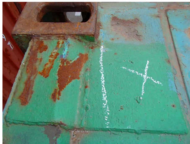
Acceptable insert on corner protection plate. Any damage to the header must have been repaired prior to insert installation.
