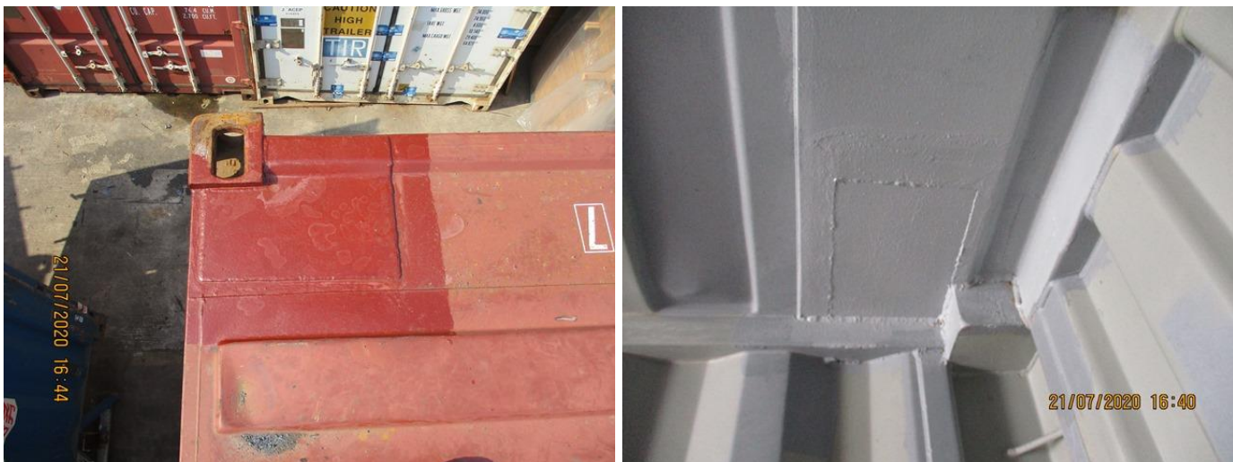
Proper replacement of the corner protection plate after installation of insert on the extension plate.
